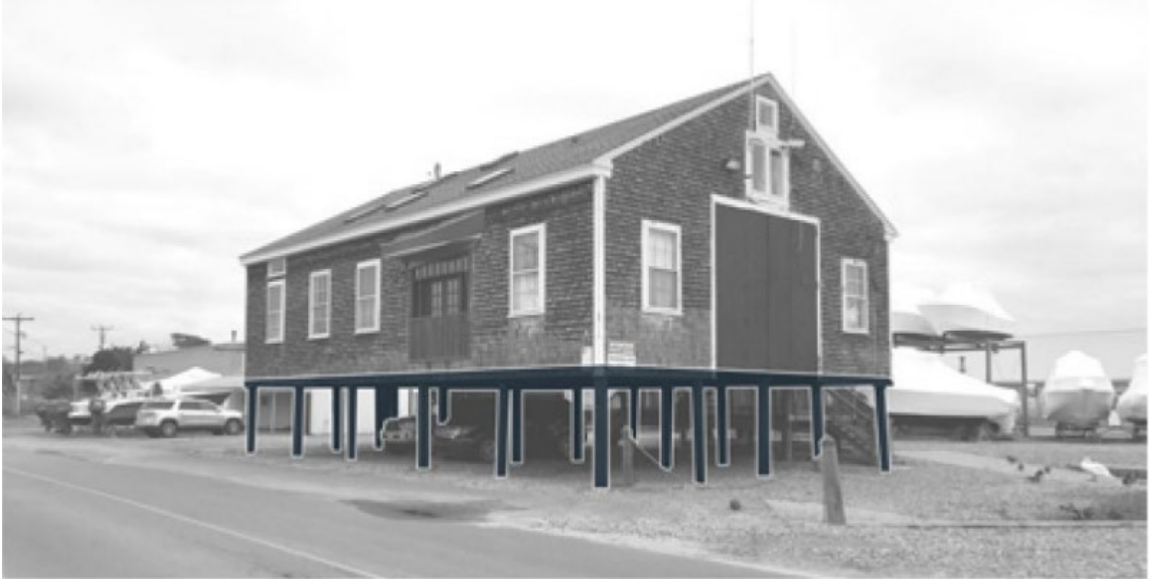
Figure C.3 Prime Marina structure at 100 Lagoon Pond Road. Some properties have begun to elevate service building in the waterfront (EPA 2020).
